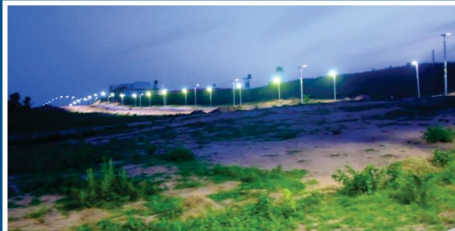
Solar-powered street lights at night - Operation Light-up Felele Campus
