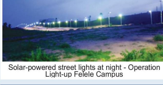
Solar-powered street lights at night - Operation Light-up Felele Campus
