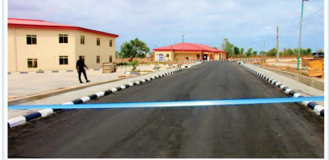
Construction of Road Network
