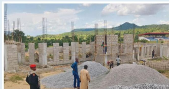
Chapel of Grace Auditorium (under construction)
