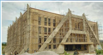
Four-storey Senate Building under construction
