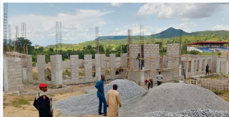
Chapel of Grace Auditorium (under construction)
