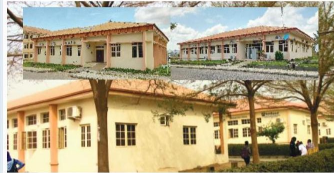
Renovated classrooms, Library, medial students hostels, ICT, and other buildings at the COHS, Adankolo
