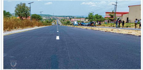
Construction of Road Network
