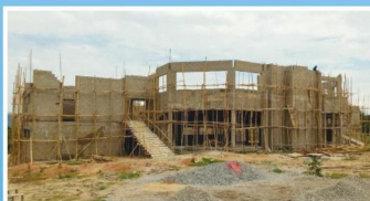
Assembly Hall (under construction)
