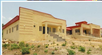
University Health Center at the Permanent Site (Phase 1 & 2)
