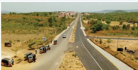
Construction of Road Network
