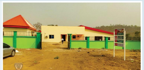
Agribusiness Incubation Centre/Cassava Processing Factory Constructed by the Fed. Ministry of Agric. & Rural Dev. (FMARD)
