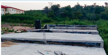
An ongoing project
