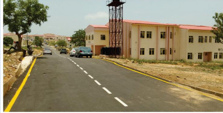
Construction of Road Network
