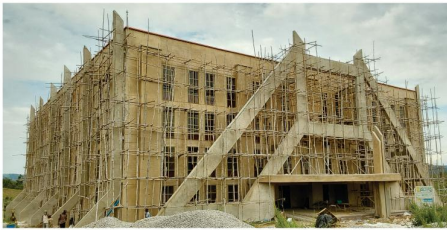
Four-storey Senate Building under construction
