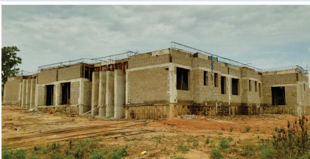
Faculty of Law Building (under construction)
