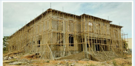
An Auditorium (under construction)
