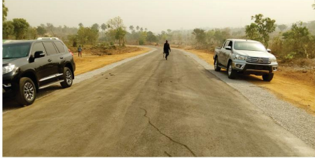
Construction of Road Network
