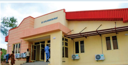
Security building with watch tower
