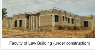
Faculty of Law Building (under construction)
