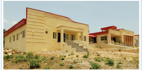
University Health Center at the Permanent Site (Phase 1 & 2)
