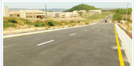
Construction of Road Network
