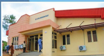
Security building with watch tower
