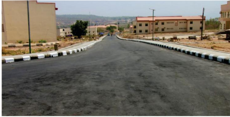
Construction of Road Network
