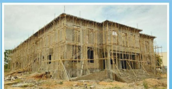
An Auditorium (under construction)
