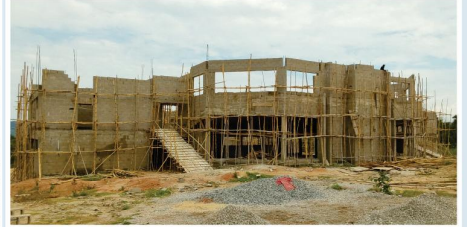
Assembly Hall (under construction)
