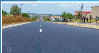
Construction of access road from the main gate
